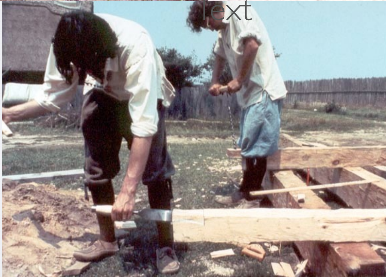
Cutting tenons on studs
